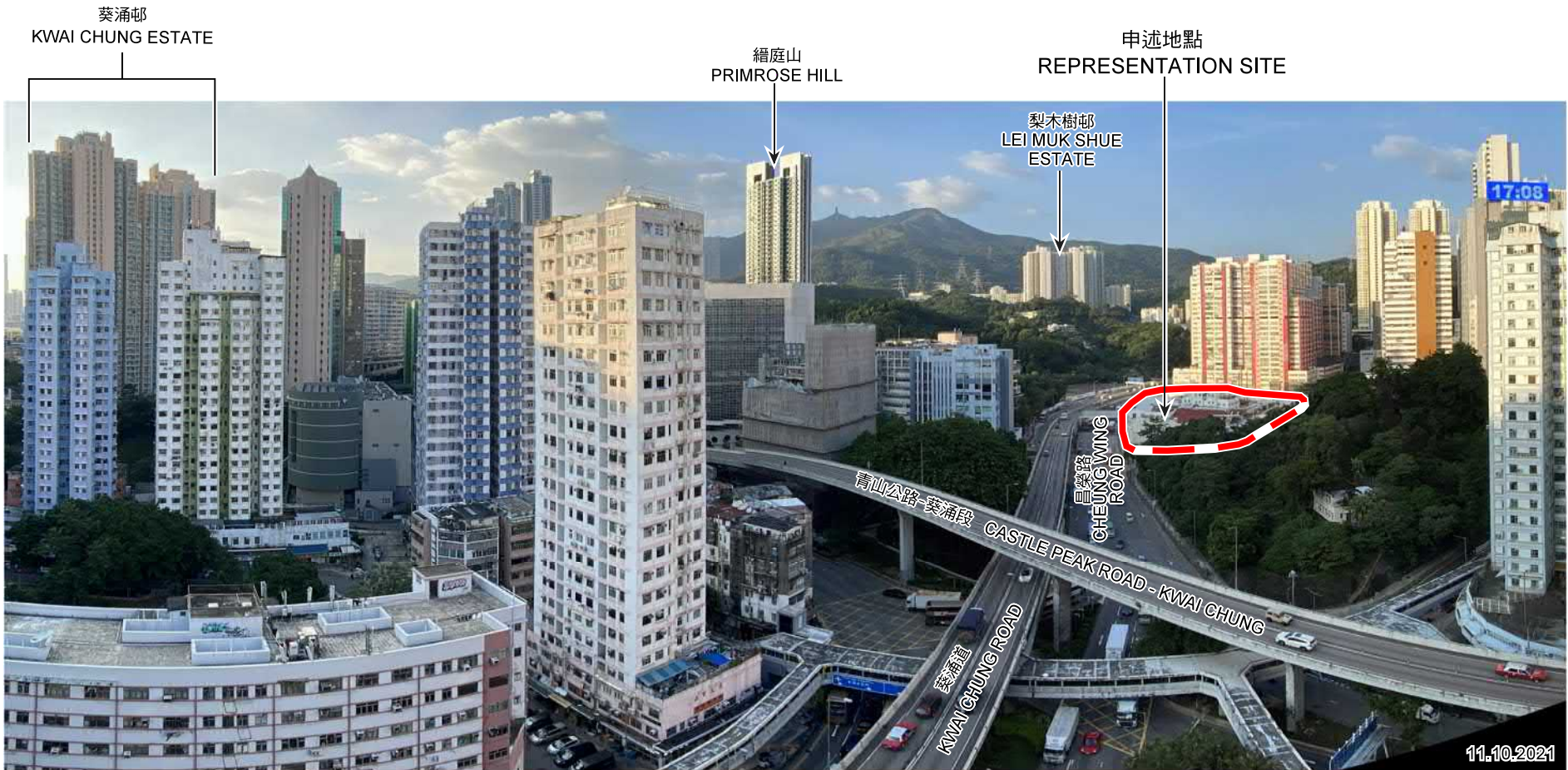
由南面觀望的景觀 VIEW FROM THE SOUTH
