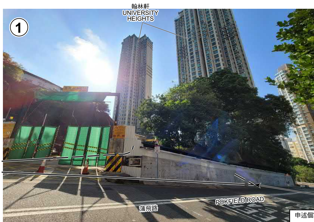
Photo taken on 4.11.2021. Part of the building structures of the Residence have been demolished. 照片於2021年11月4日拍攝，宿舍的部份樓宇構築物已被拆除。
