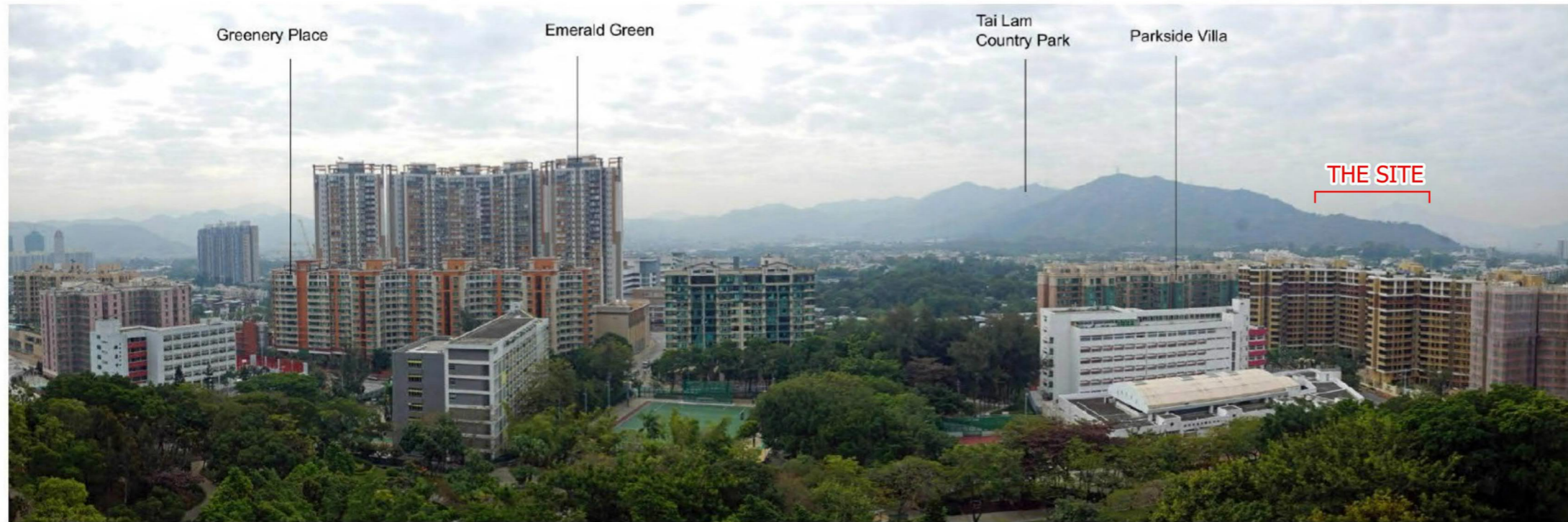
Yuen Long Park Tower - Existing View (Approx. 540m)
