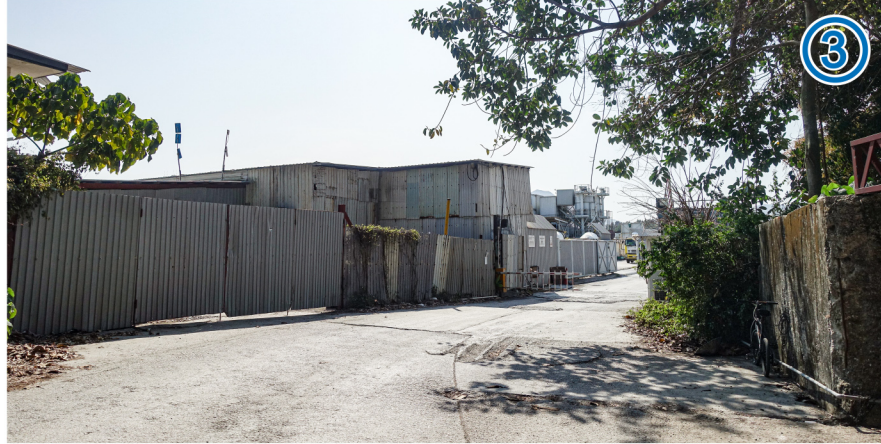
Temporary concrete batching plant approved under application no. A/NE-TKL/681
