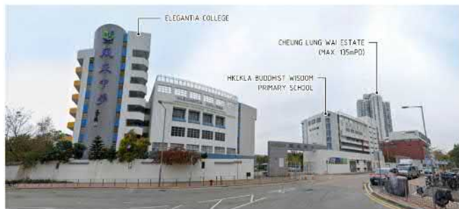
VP12 - ELEGANTIA COLLEGE - EXISTING SITE CONDITION
