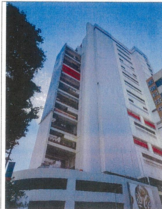
**Fig 1. Semi open-air design for upper floors**
