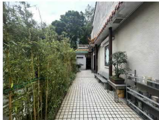
Photo 7: Bamboos along the side of Building A.
