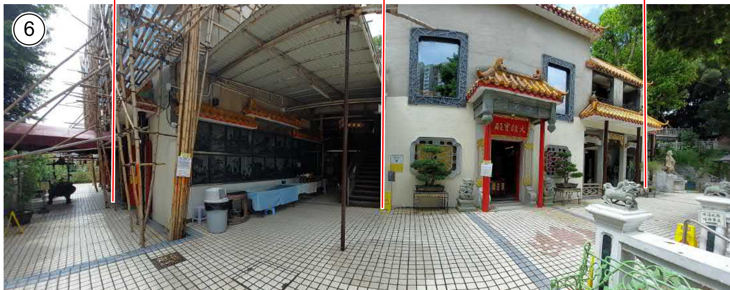
建築物A及B Building A and B
