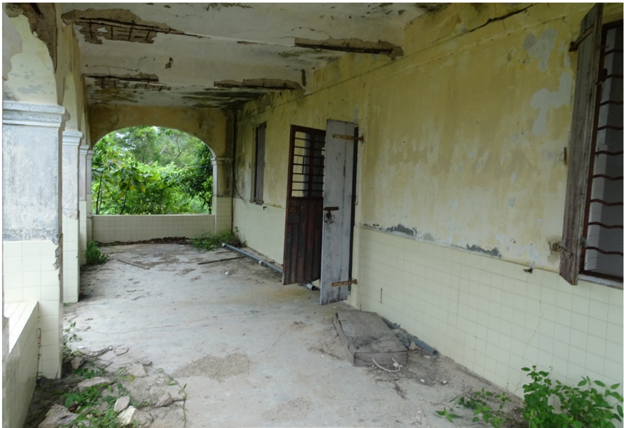
( 現有屋宇內部情況 ) ( Interior condition of existing house )
