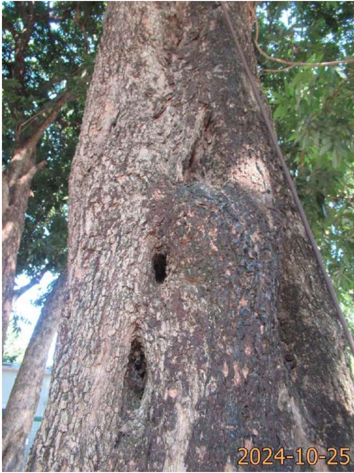
T20 Cavity at trunk
