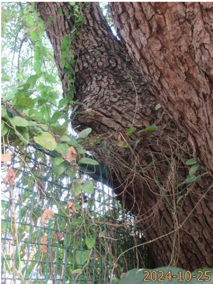
T13 Trunk conflict with fence
