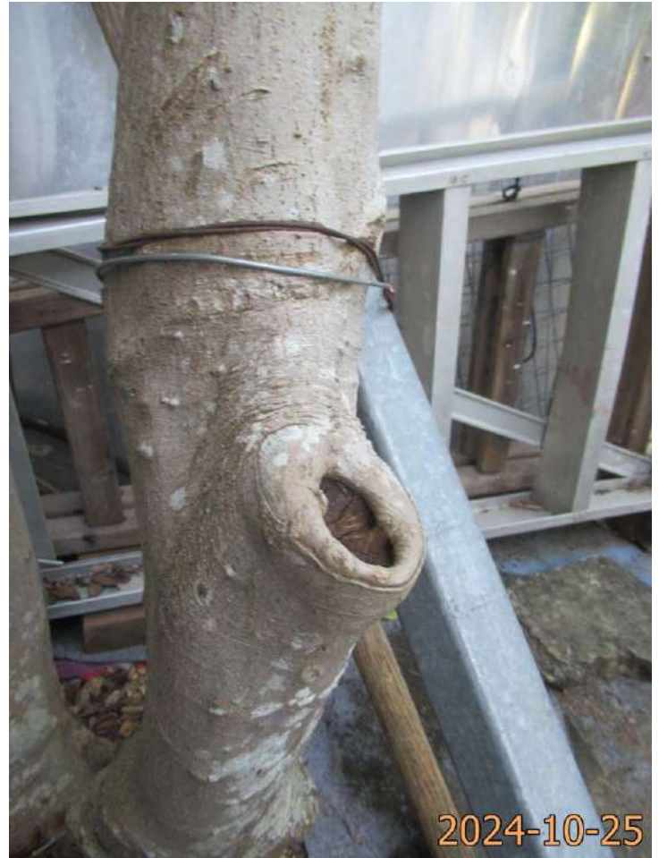
T16 Cavity at trunk
