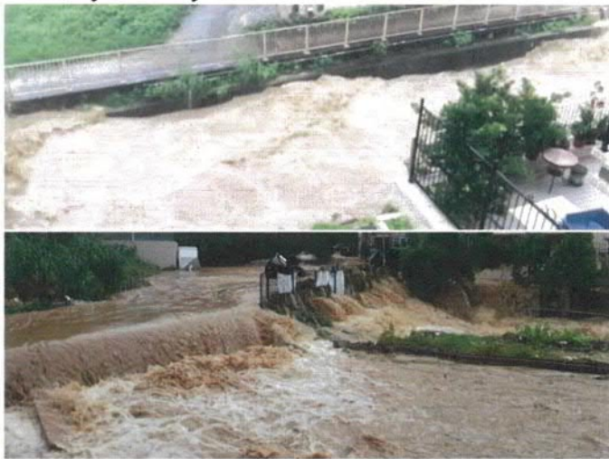
Figure 1: The flooding due to the amber rain in 2017
