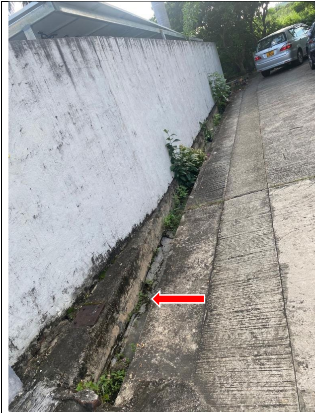
Photo No.3: Existing 300mm UC along Northern Boundary
