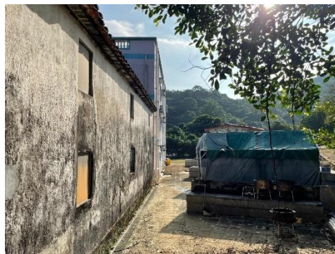
3.Vacant Land at the behind
