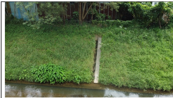
Plate 15 – Existing 600mm stepped channel discharging into Ng Tung River at the downstream of the Application Site
