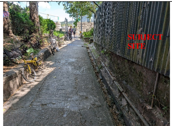
Plate 8 – Existing 300mm U-channel running between the eastern subject site boundary and an existing external footpath (1 of 3)
