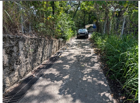
Plate 6 – Existing 450mm U-channel running westward along the existing access in front of the southern subject site boundary (2 of 2)
