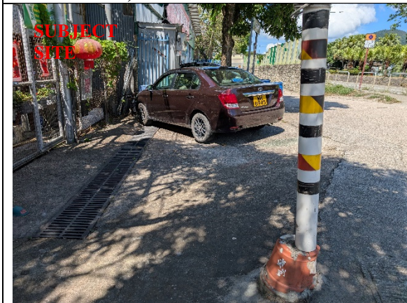
Plate 7 – Existing 450mm U-channel running eastward along the existing access in front of the southern subject site boundary
