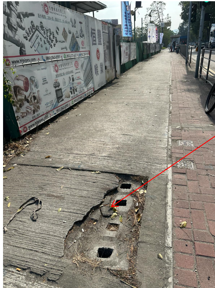
VIEW 1 1m(W) x 1m(H) underground channel
