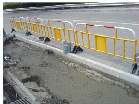
(4) Concrete paving
