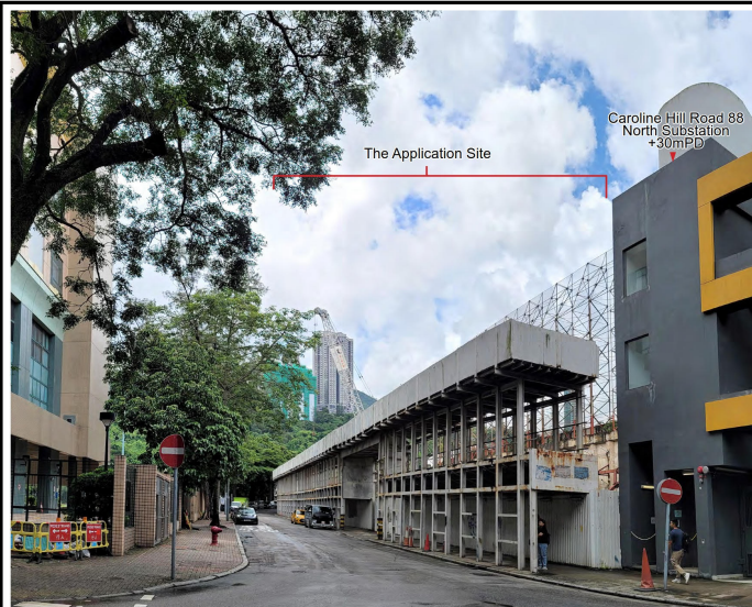
Existing View View southeast from the junction of Caroline Hill Road & Cotton Path
