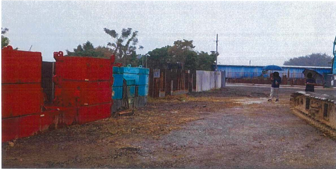
Photo V9 - General view of the site
