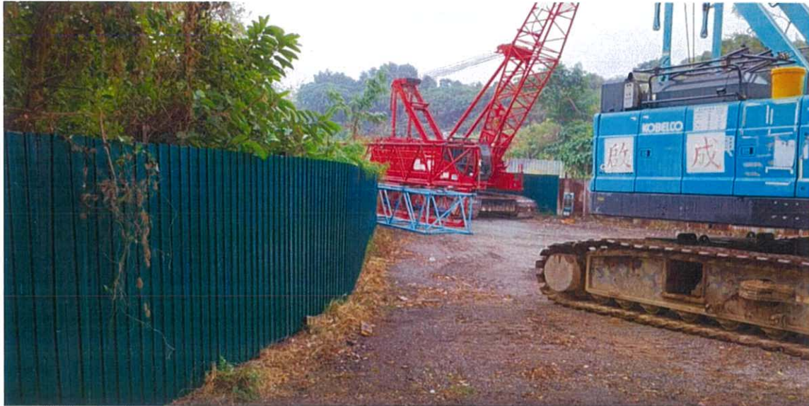
Photo V7 - General view of the site
