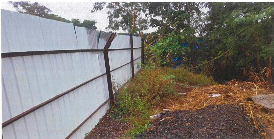
Photo V4 - General view of the site
