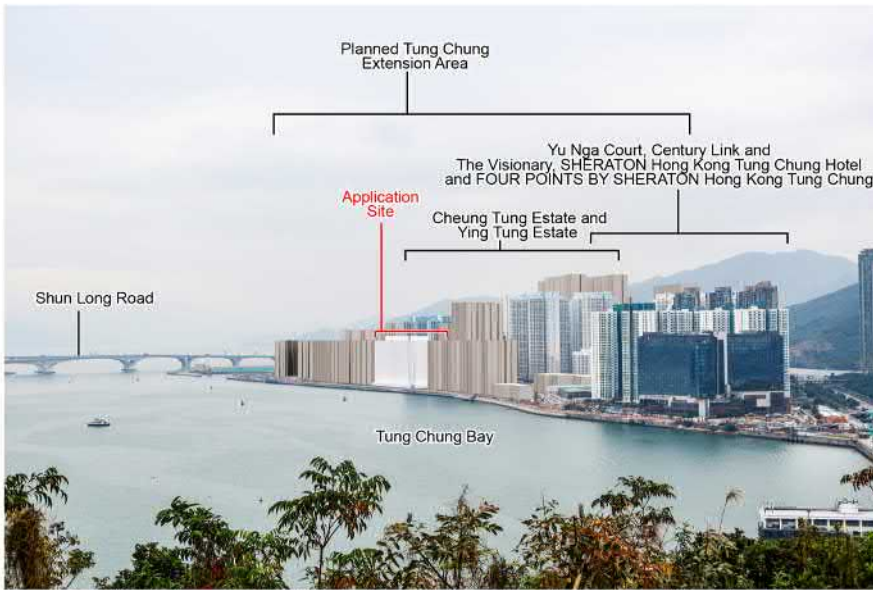
Approved GBP Scheme – After the Implementation of the Tung Chung Extension Area
