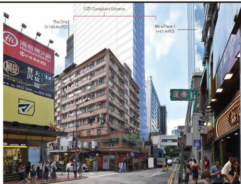
Vantage Point 01: View looking south west from the j/o of Kimberley Road and Carnarvon Road (OZP Compliant Scheme)
