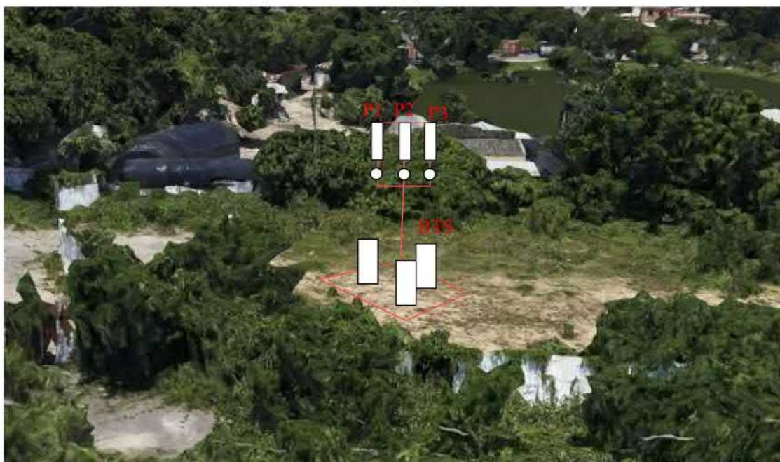
Photo 3: Proposed concrete plinth for BTS equipment and antenna posts P1 to P3 location
