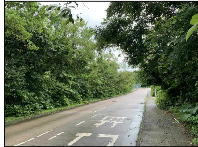
EXISTING PHOTO PHOTO DATE: 24/09/2024
