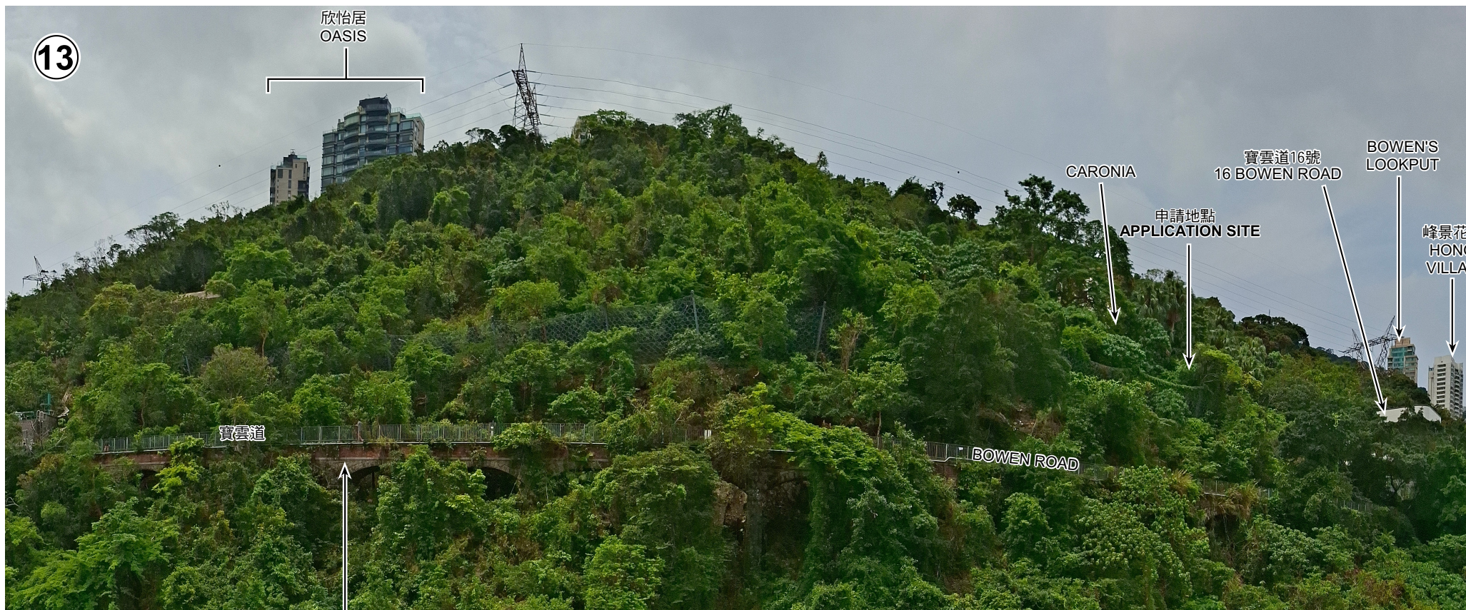
寶雲道21孔拱券段 21-ARCH SECTION OF THE BOWEN AQUEDUCT
