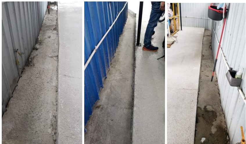
Photo 7: Series showing the 300mm open channel along the site boundary
