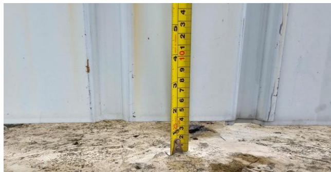
Photo 8: Minimum 30mm spacing for water flow underneath of hoarding
