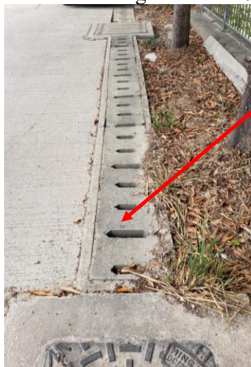
Photo 1: Roadside existing U-Channel
