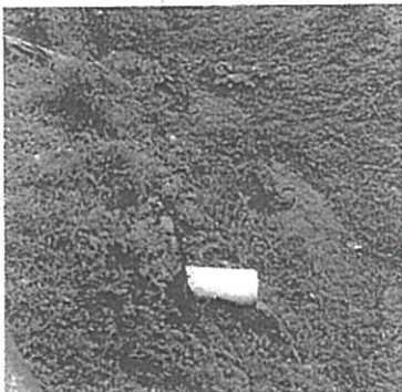
Existing outfall for gully
