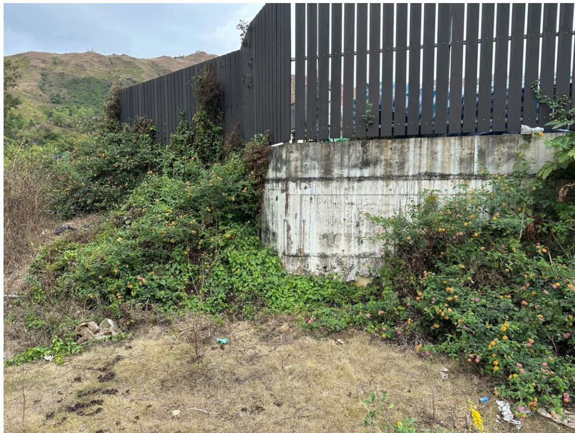
Photo 2: Concrete Footing at the Site Located at the North of the Project Site
