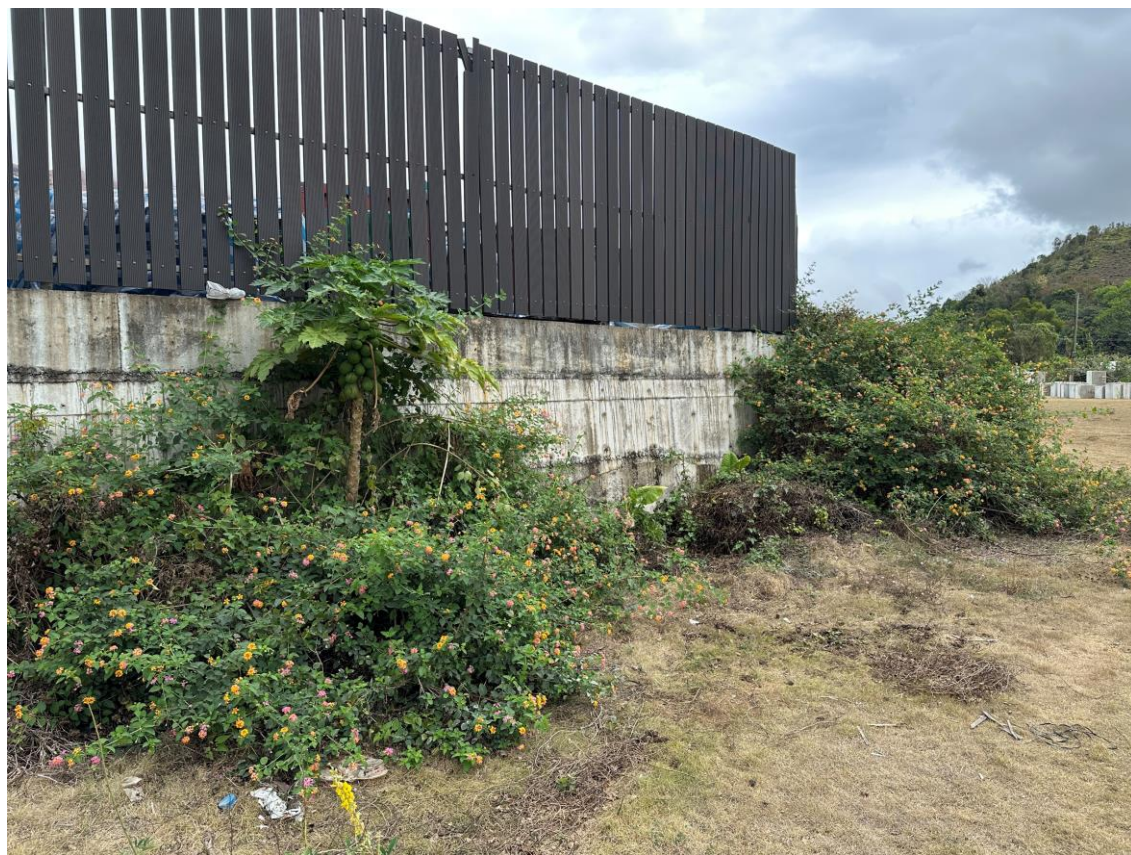
Photo 1: Concrete Footing at the Site Located at the North of the Project Site
