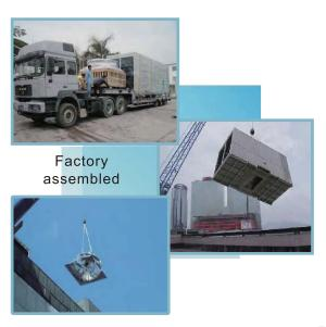
Most FWS cooling towers can be factory assembled and delivered to site.
