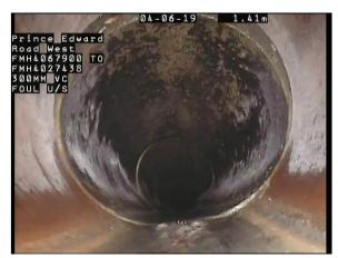
0001, 0:00:47 Crack Circumferential AT Joint, from 10 to 05 o'clock Video Tape : Observation :
