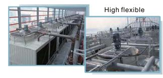
All FWS models can be fitted with RYOWO special integrated drift eliminators to achieve drift loss less than 0.001% and equipped with OSHA handrail and caged ladder to comply with requirement.
