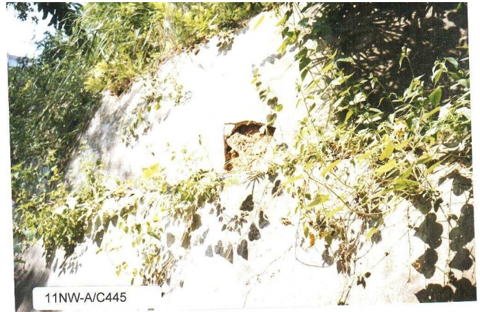
Missing chunam above the beam.
