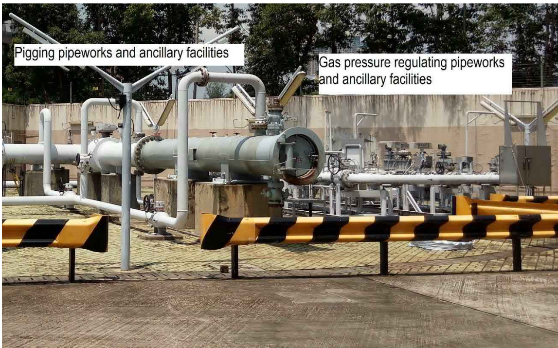
(b) Aboveground Gas pressure regulating/Pigging pipeworks and ancillary facilities
