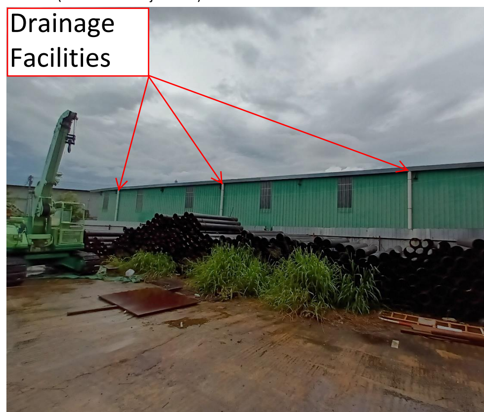
Photo B - Concrete Surface of Subject Site and Drainage Facilities of Lot 1264 S.A in D.D. 124 (West of the Subject Site)
