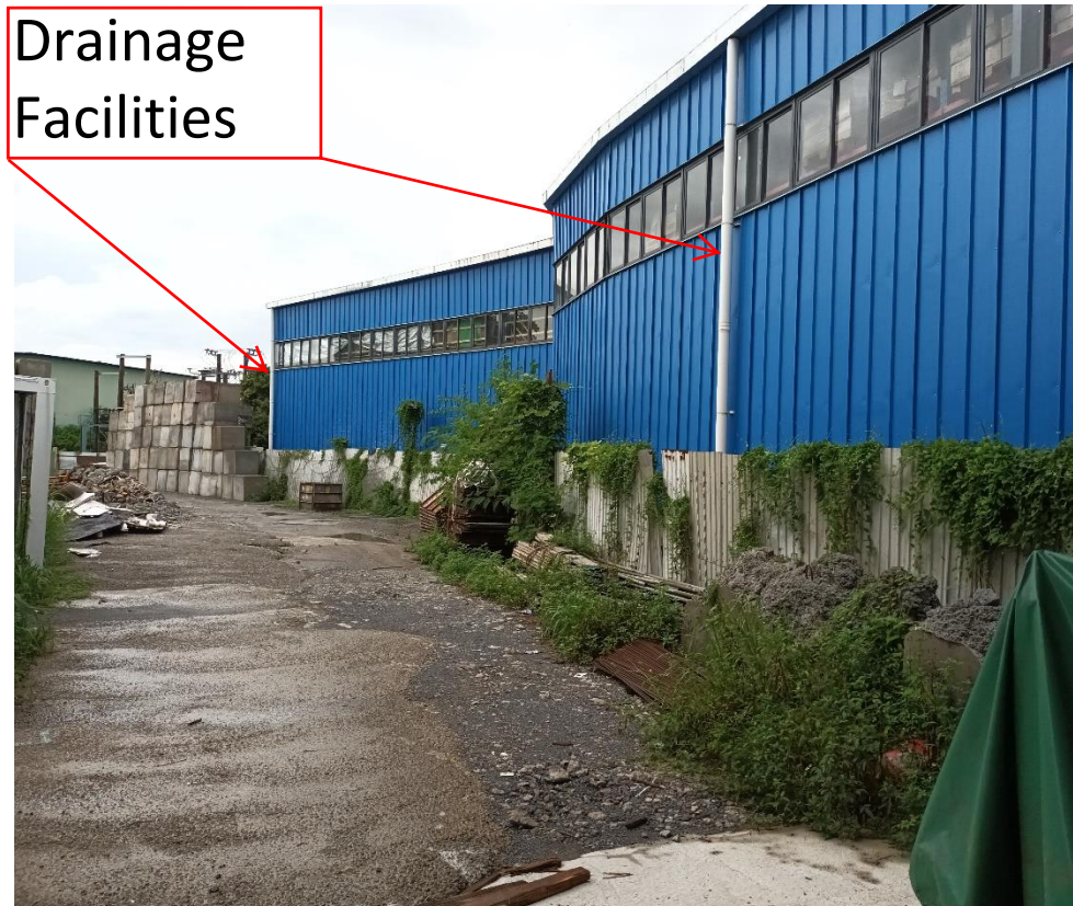
Photo A - Concrete Surface of Subject Site and Drainage Facilities of Lot 1261 in D.D.124 (East of the Subject Site)
