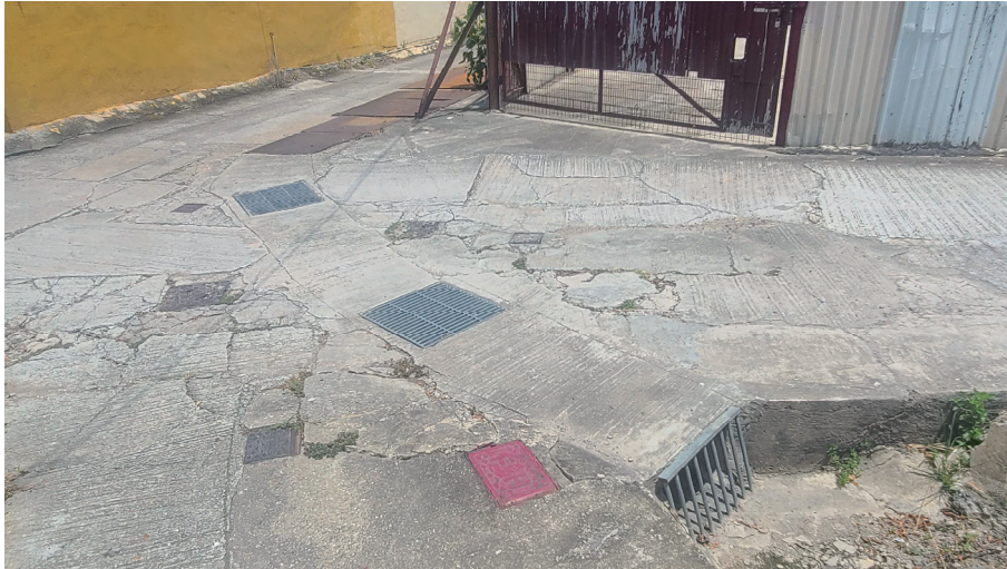
Plate 1 – The inlets of the existing 600UC
