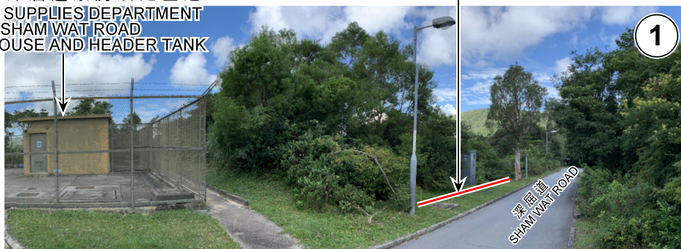
水務署深屈道泵房及定壓池 WATER SUPPLIES DEPARTMENT SHAM WAT ROAD PUMP HOUSE AND HEADER TANK
