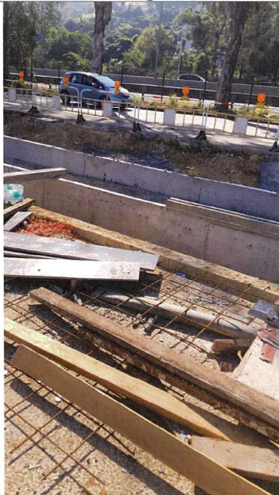
View 2 “ Existing Nullah” removed and reconstructed to 750UC
