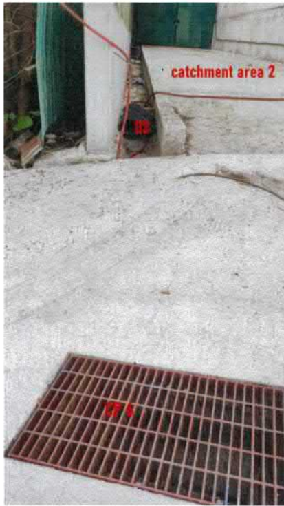
fig 1 Catchment Area 2, D3 and CP6 with metal grille, on left is neighbouring site at downstream and has its own drainage
