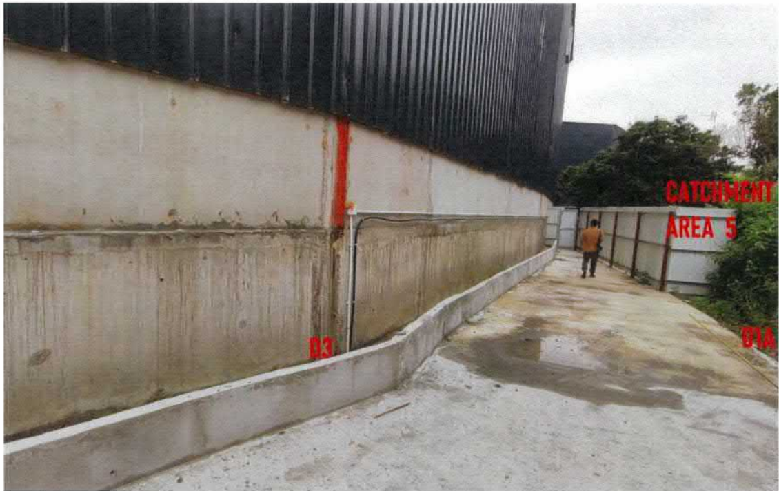
fig 6 Northern edge of Site, with Catchment Area 5 (on right, North). D3 is to collect the runoff of Site (temporary structure). D1A to collect runoff from Catchment Area 5.
