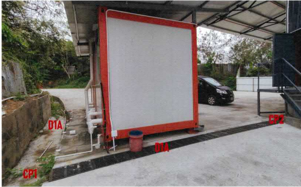
fig.4 D1A collect runoff of slope of left (Catchment Area 5) and discharge via CP1/CP2 to CP3; CP3 will also carry discharge of part of Roof Structure (Catchment Area 1)
