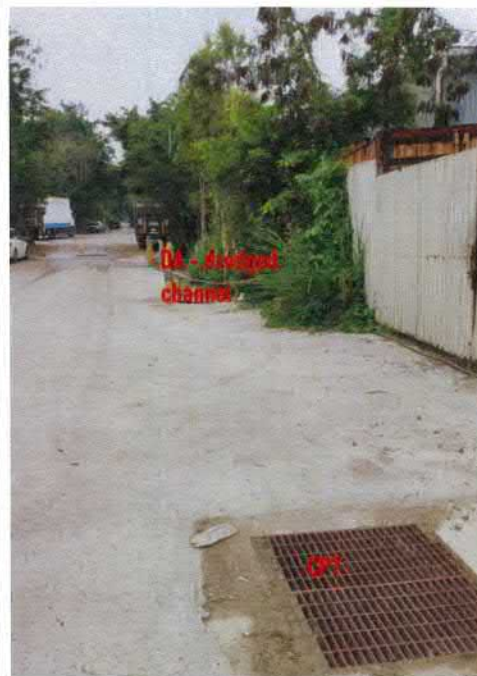
fig.3A CP7 and underground drainage pipe to discharge to village channel DA
