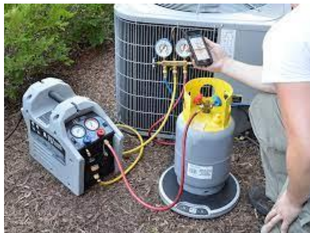
Figure 3. Application of refrigerant recycle system on chillers
