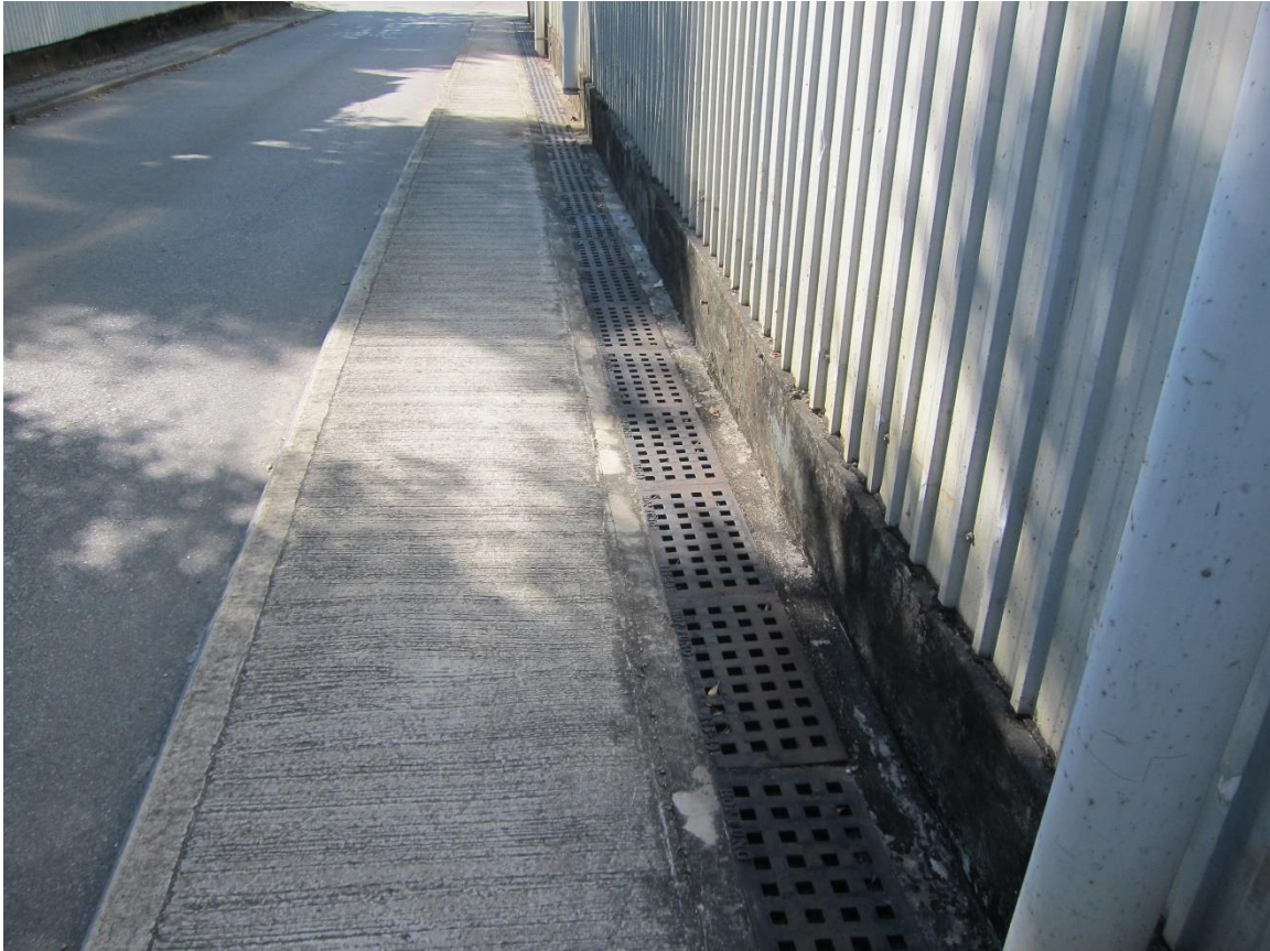
Photo 4: Existing u-channel on the ground
