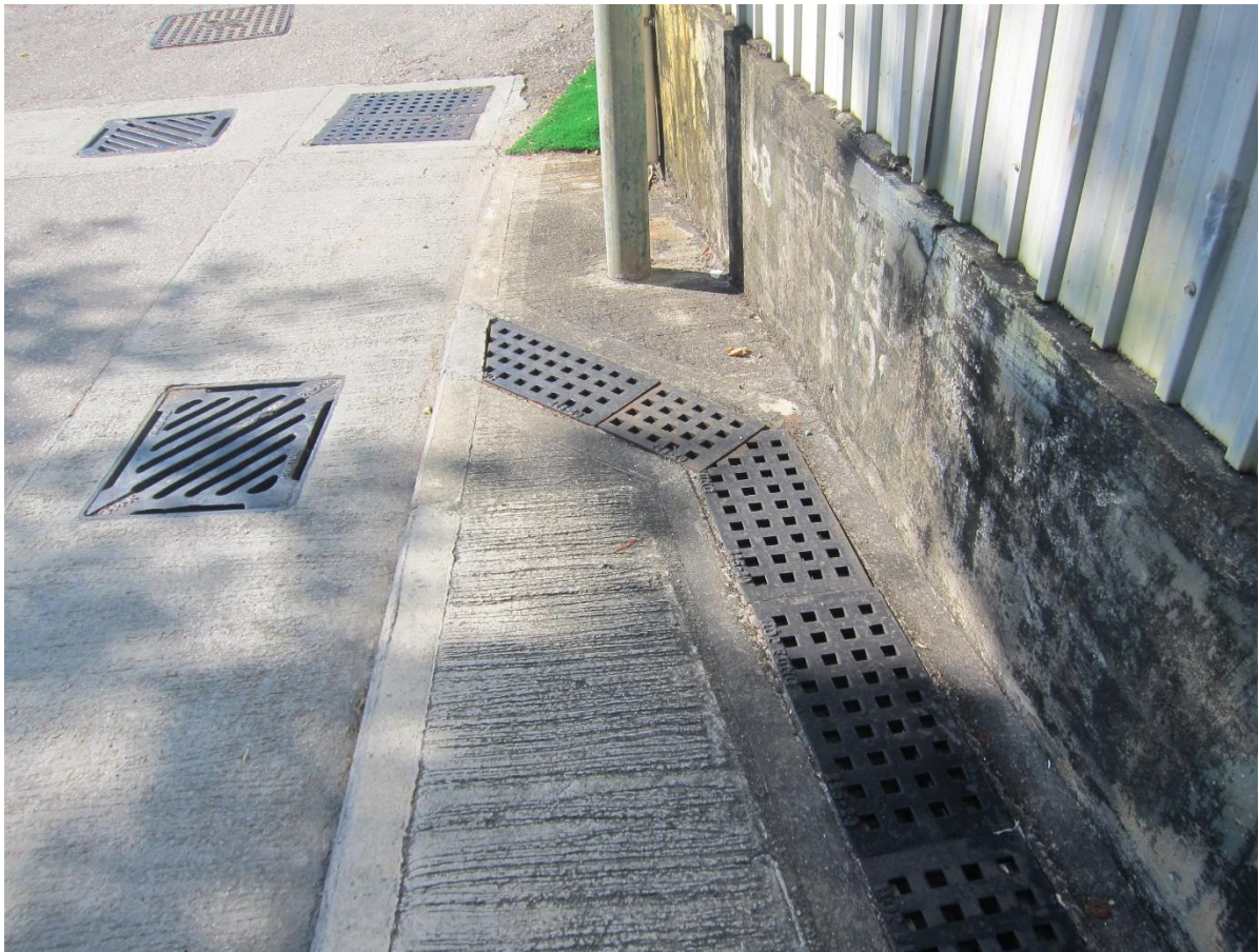
Photo 5: Existing u-channel on the ground
