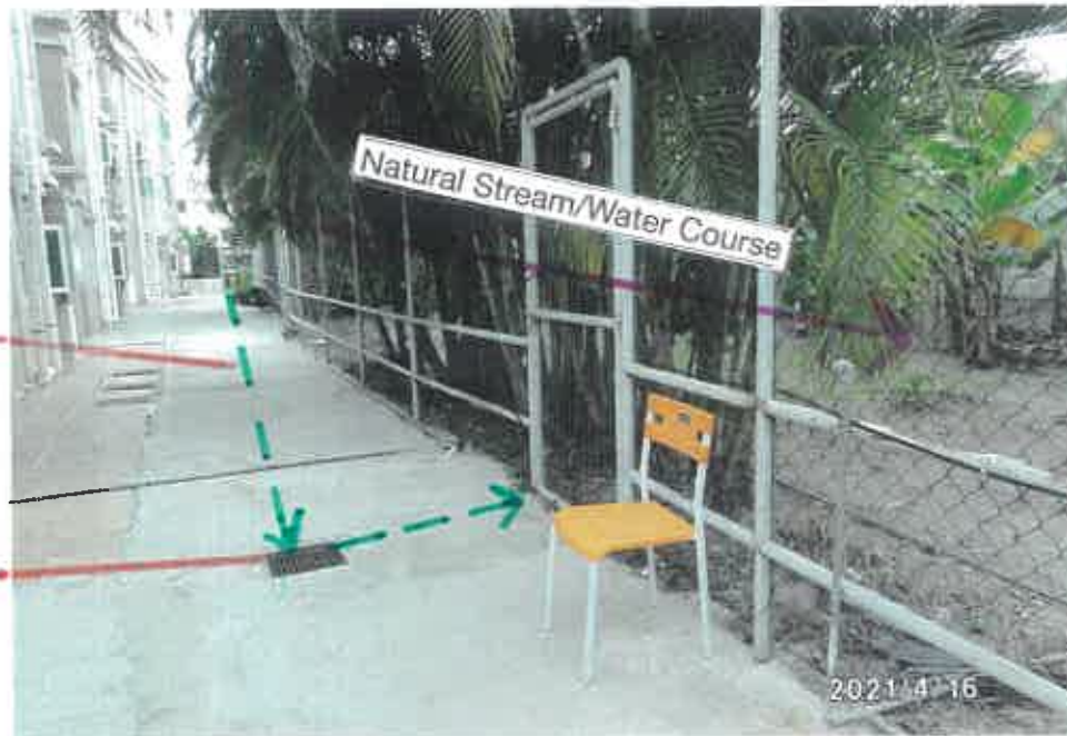
Grating 6. Underground drain
