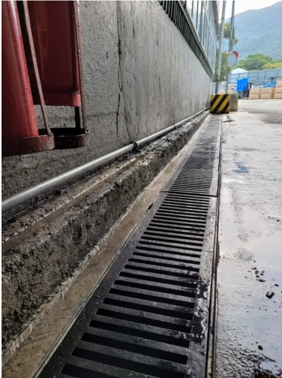
Photo 13: Existing 600 U/C Condition
