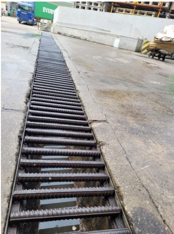
Photo 9: Existing 225 U/C Condition
