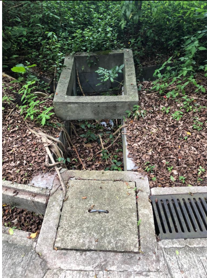
View 1 Existing 225UC and Catchpit
