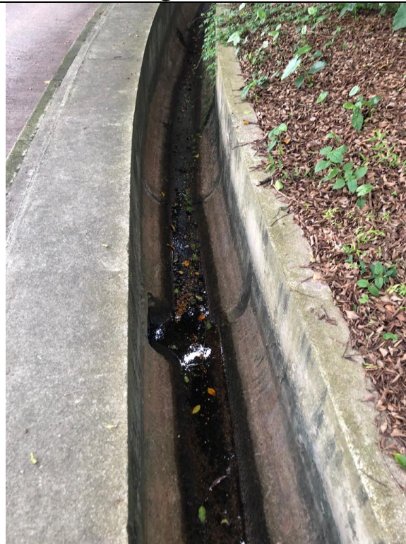
View2 Existing 600UC within 300x 300 underground drain
