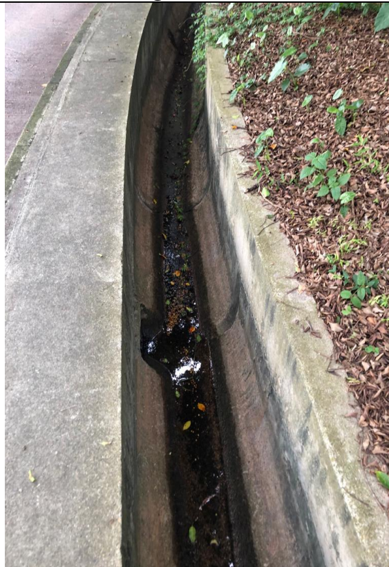
View2 Existing 600UC within 300x 300 underground drain
