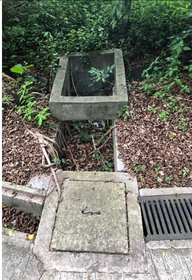
View 1 Existing 225UC and Catchpit
