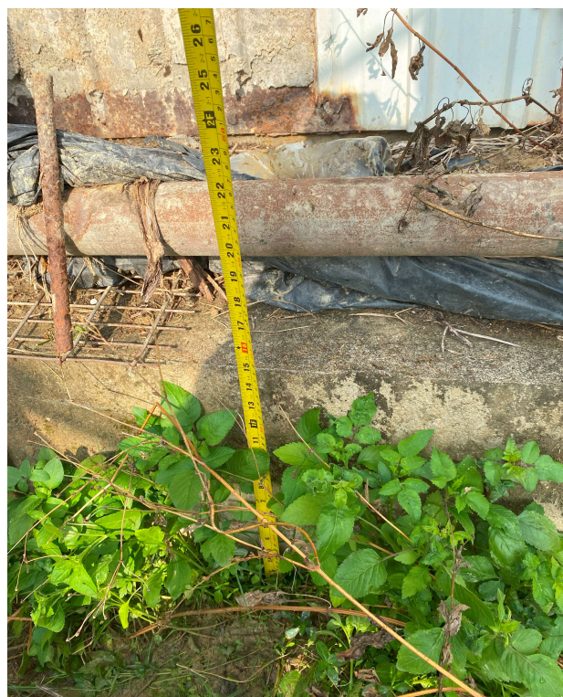
Photo View: A8 (The concrete channel is around 380mm deep)
