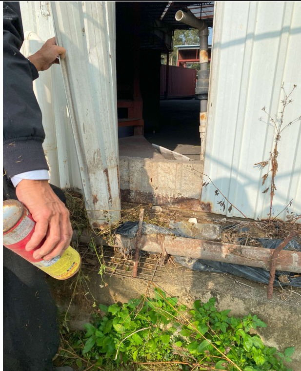
Photo View: A7 (Corrugated sheet was cut to verify the condition of "Retaining Wall")
