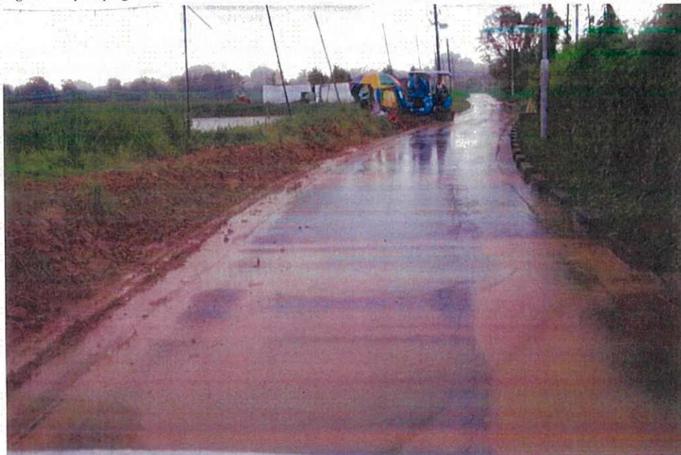
Figure 3. Pipe-laying works within the CA zone near Mai Po involving excavation of a trench; muddy runoff generated under heavy rain.
