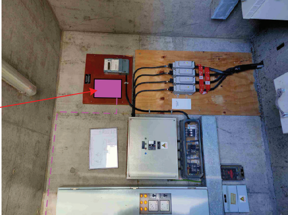
NEW 60A SPN CLP ELECTRICITY METER IN SWITCH ROOM NO. 6
