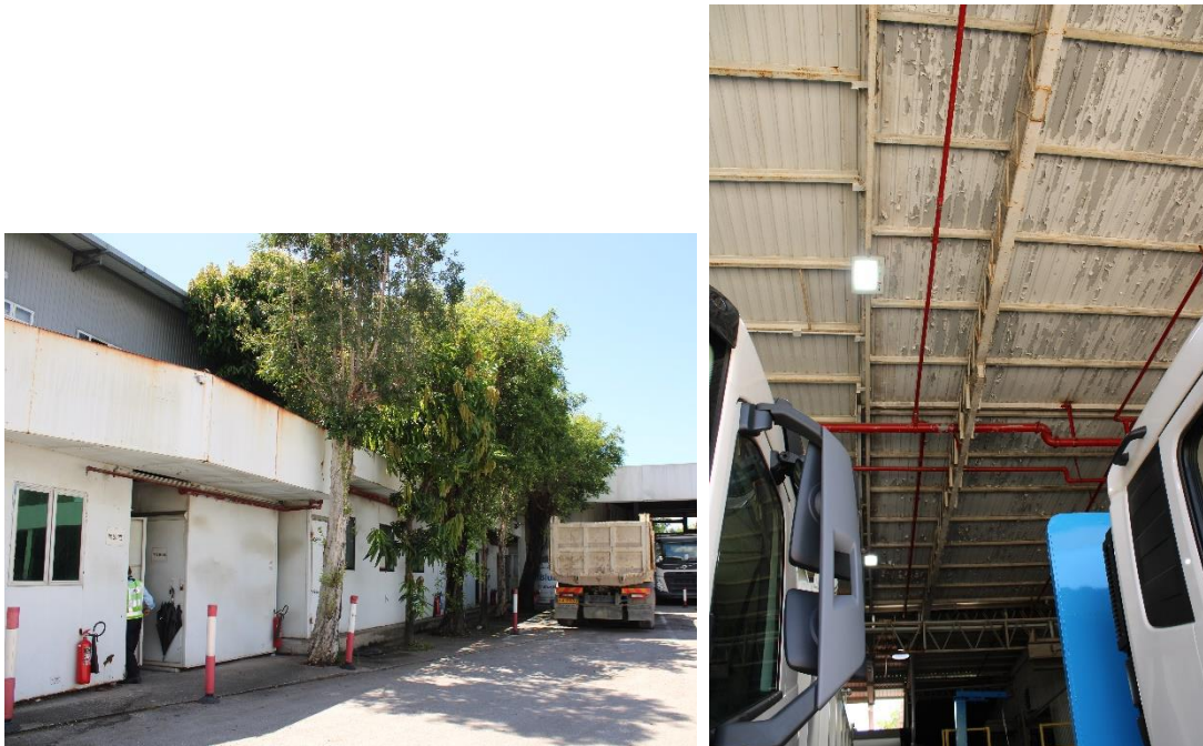
Photos 3.1 (Left) and 3.2 (Right): The Existing Fire Extinguishers and Automatic Sprinkler System
