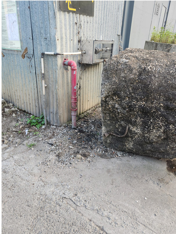
Water Supply for Fire Service Tank
