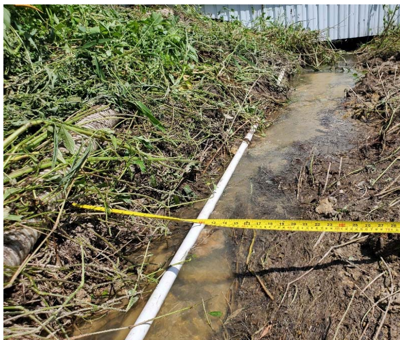
Existing drainage system, 450mm trench
