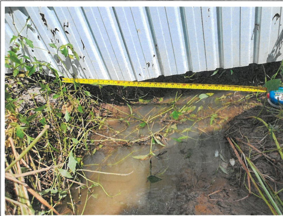
Photo 6- Existing drainage system, 450mm trench
