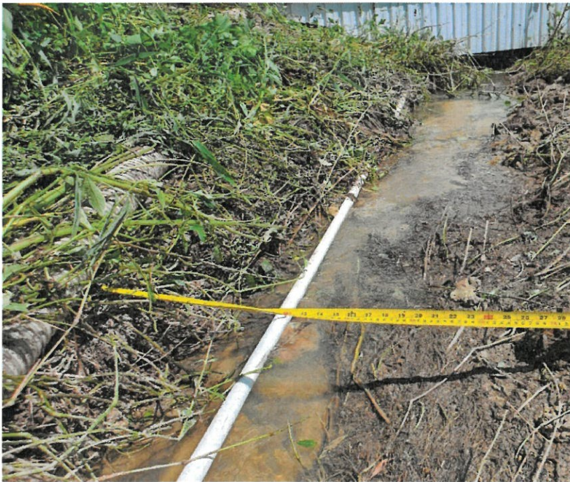
Photo 2- Existing drainage system, 450mm trench
