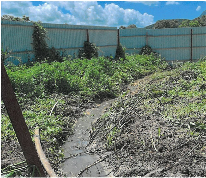
Photo 1- Existing drainage system, 450mm trench
