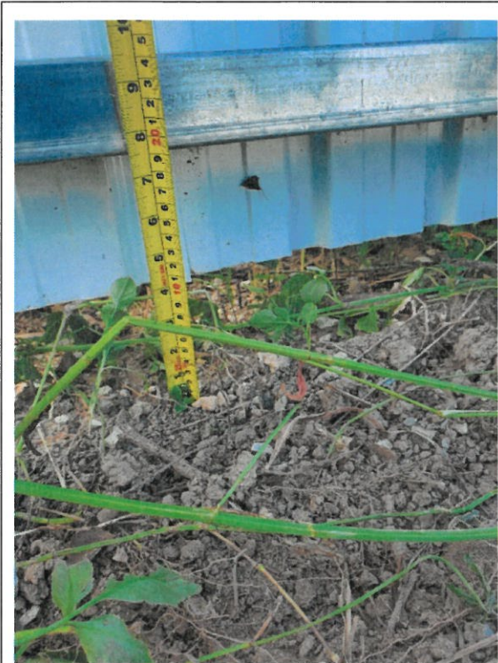
Photo 3- Sufficient openings (100mm) provided at the bottom of boundary wall/fence to allow surface runoff to pass through the site
