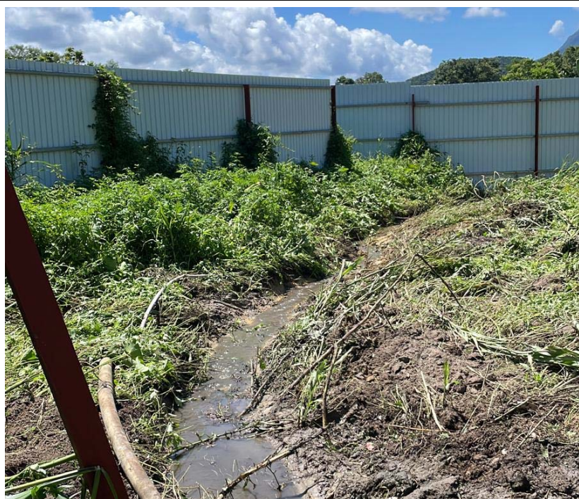
Existing drainage system, 450mm trench
