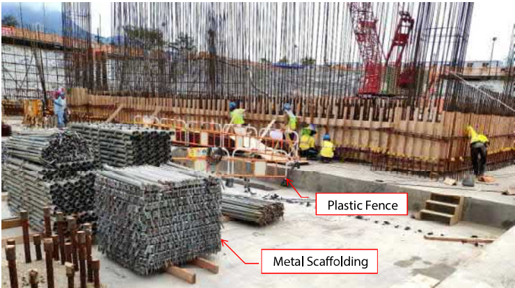
Stage 3– Substructure Works
