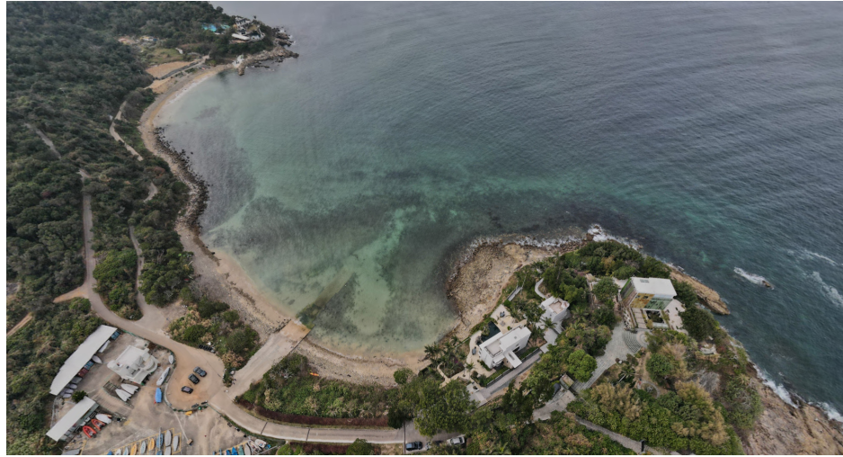
Figure 4.5.3 Existing condition at the surrounding of the site 2
