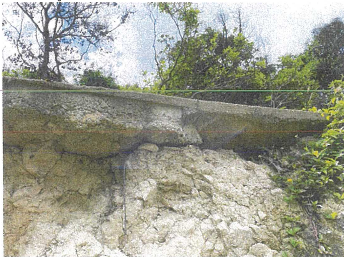
Photo 2: One of the sections of the paved road connecting between the application site and the Hang Hau Wing Lung Road
