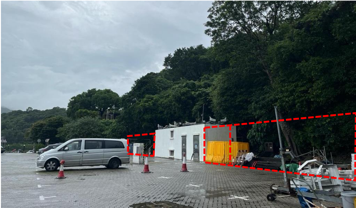
Photo 1: Location of the both the proposed 1 storey buildings for ancillary use. The staff office is on the left of the existing electric sub-station (structure painted white in the centre), and refuse collection point and storage facilities on the right.
