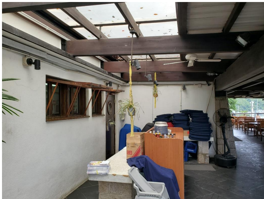
Photo 4: Existing situation outside of the kitchen, where the serving area is partly occupied as storage space.
