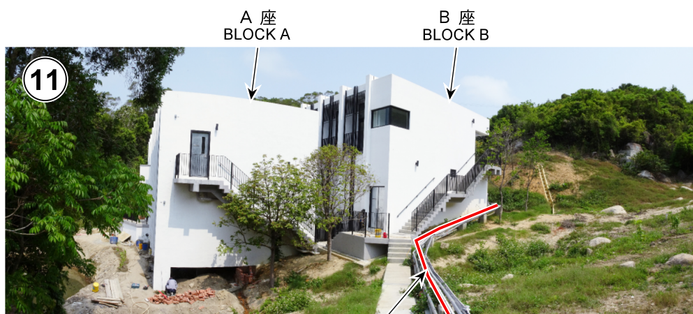
管道 UTILITY PIPE
