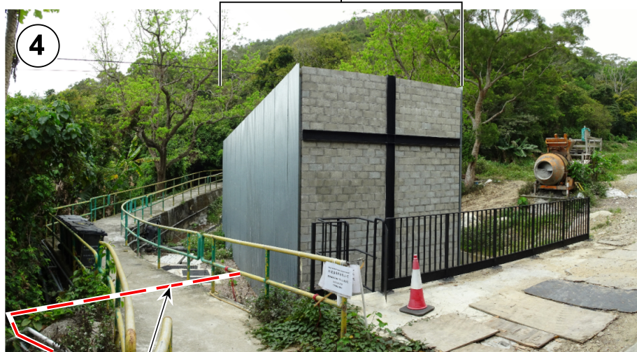
管道 UTILITY PIPE
