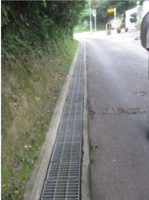
Photo 3 Existing 375mm surface U-channel along the slope
