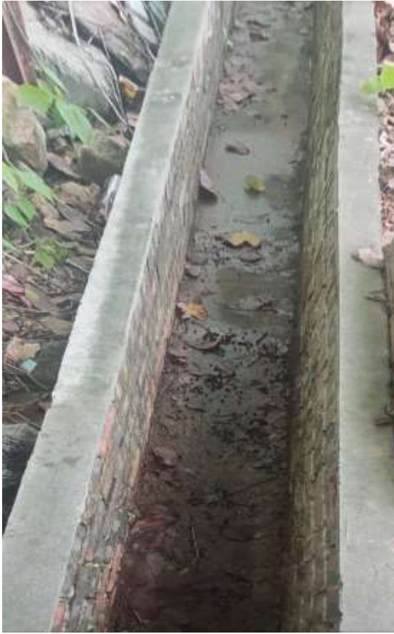
Photo 2 showing the existing 375mm surface U-channel
