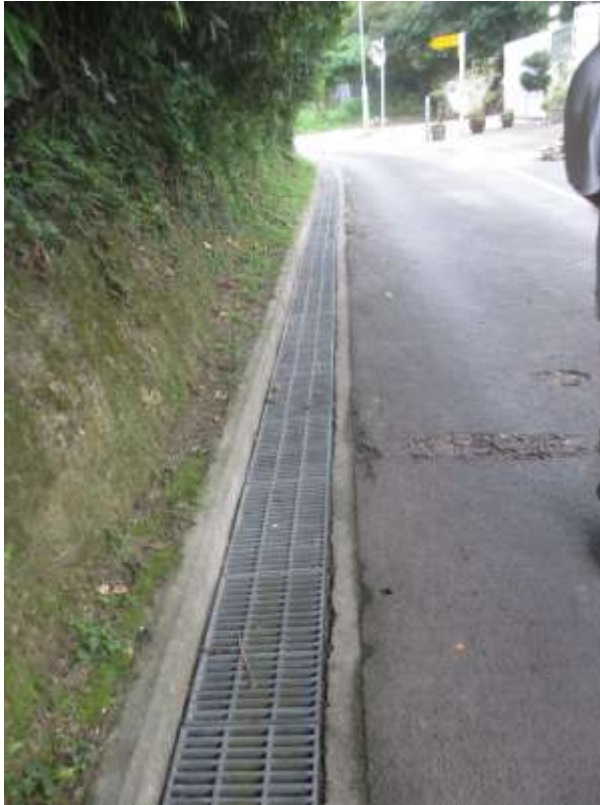
Photo 3 Existing 375mm surface U-channel along the slope
