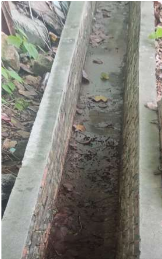
Photo 2 showing the existing 375mm surface U-channel
