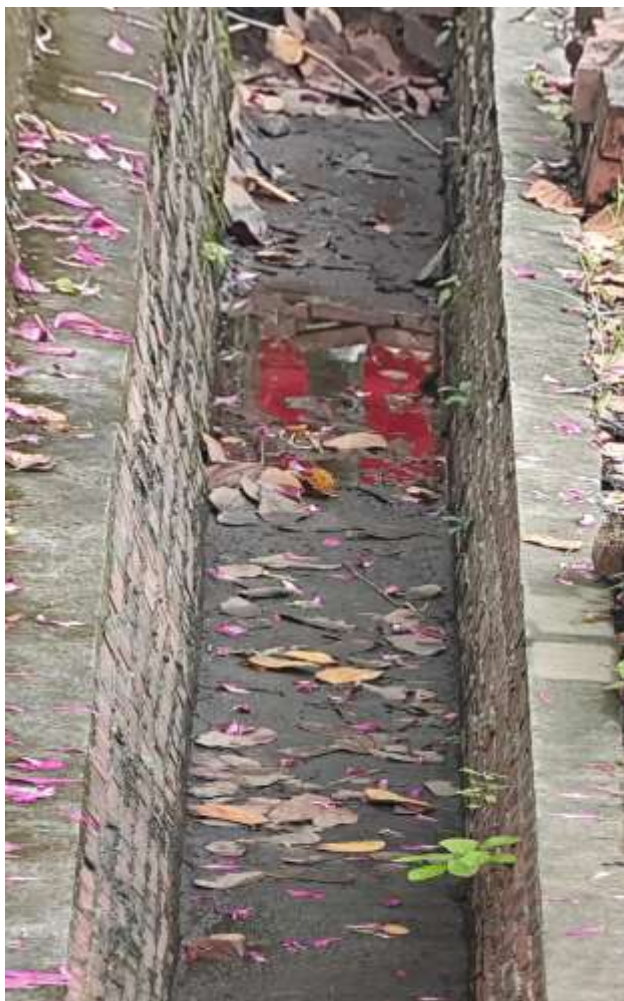
Photo 2 showing the existing 375mm surface U-channel
