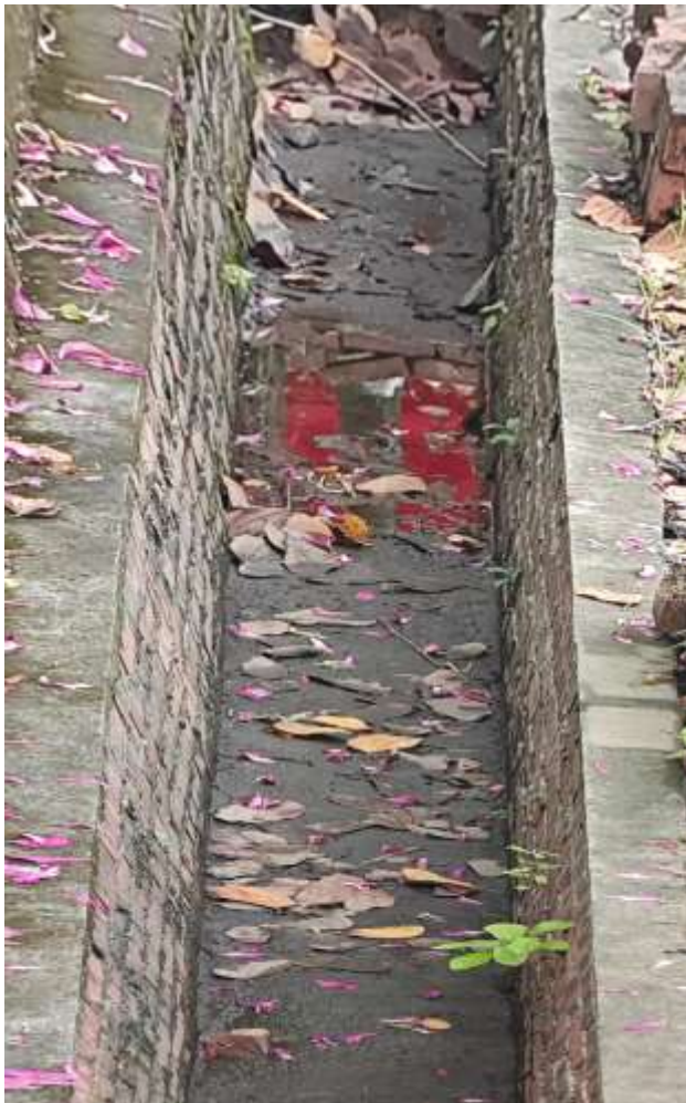
Photo 2 showing the existing 375mm surface U-channel
